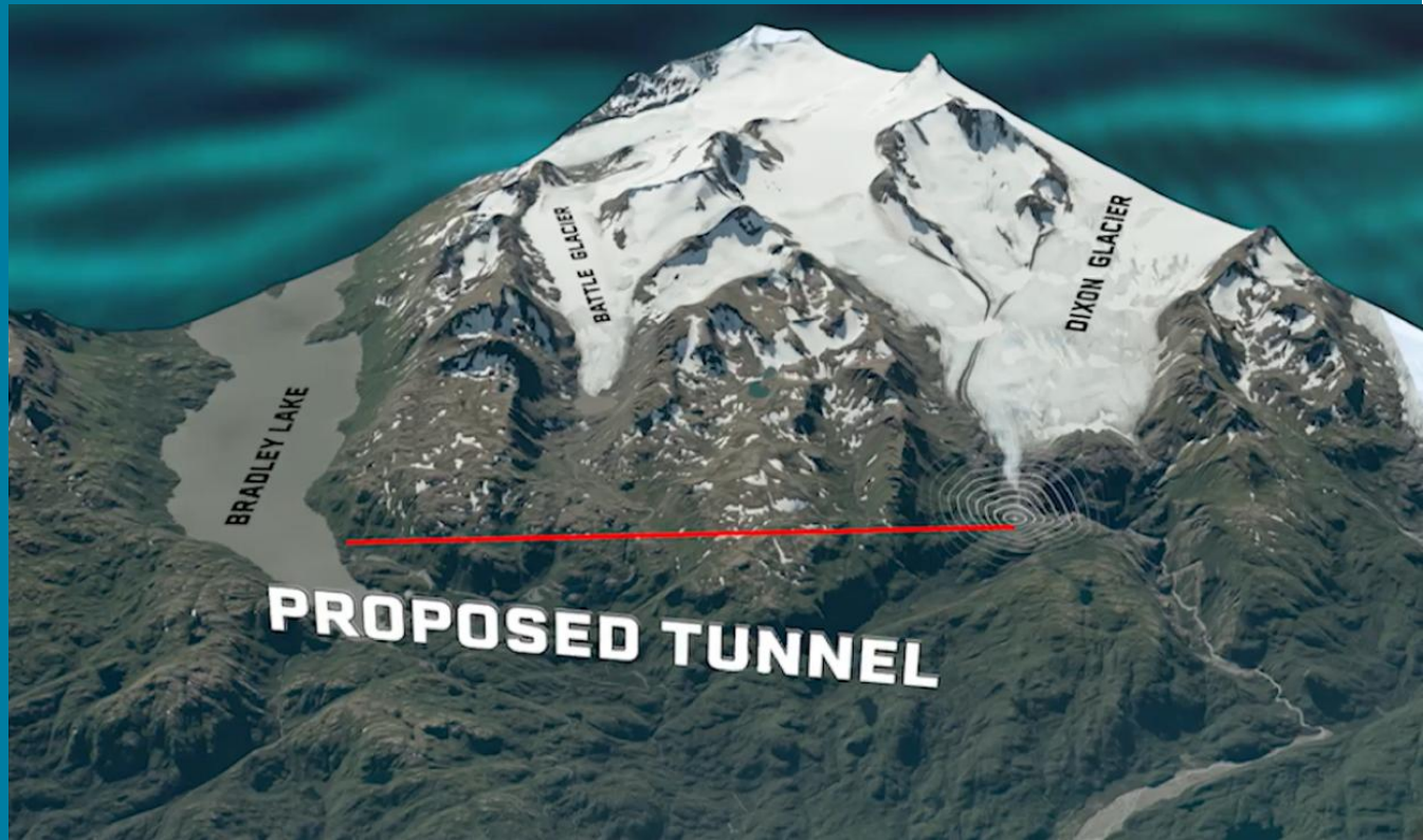
Dixon Diversion: 4.6-mile tunnel routing water from Dixon Glacier into Bradley Lake.
